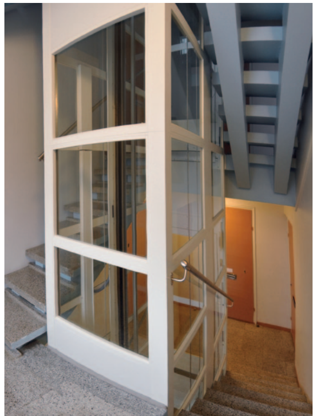
The KONE Motala 6000 elevator is self-supporting, so it puts no stress on the building walls.
